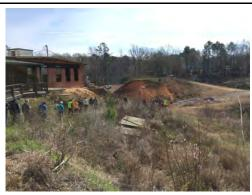
Old Mill Dam in Lexington, SC along Twelvemile Creek. Scour along the left abutement of the earthen embankment and Old Mill Brewpub resulted in failure of the dam during the flood. The town would like to reconstruct the dam; however, budget and funds are determining the cost and timeframe of when reconstruction will commence.
