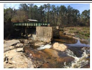
Gibson Pond Dam in Lexington, SC, along Twelvemile Creek. The concrete spillway gate structure and bridge are all that remain after the flooding event. Plans to reconstruct the dam are underway.
