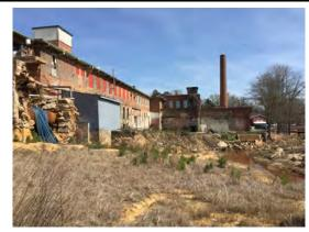
Flood damage to the Old Mill Brewpub along the left abutment of the dam resulted in structural damage to the first floor of the building, which has since been fixed, and sadly many beer kegs were swept away in the floodwaters.
